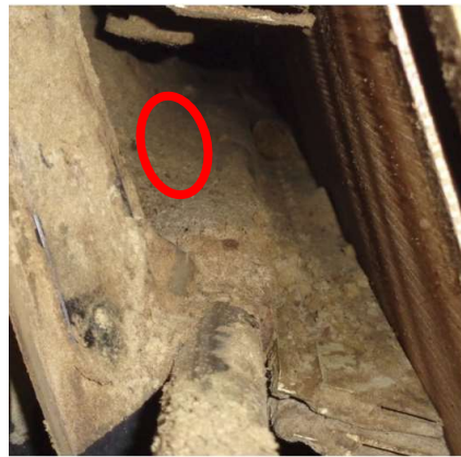
Figure 5b. Plugged suction openings
